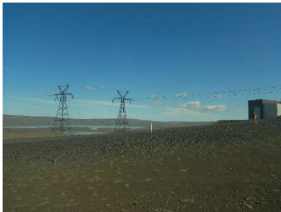
a. Power lines
