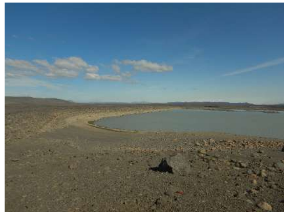
d. Hydro reservoirs and dams
